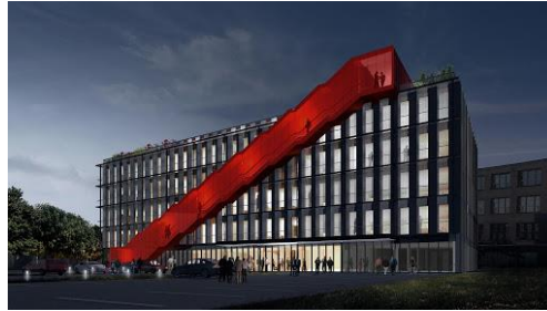
Office building RED-LINE Riga, Latvia
